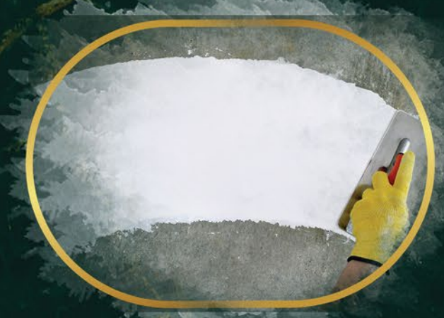
Internal wall Finish – Wall putty
